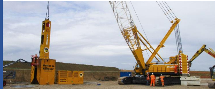
A representative image of test piling works
