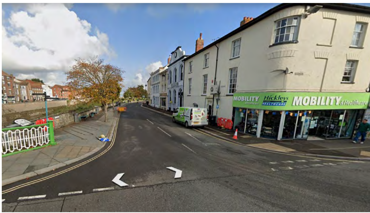
VIEW 04: TOWN BRIDGE LOOKING NORTH DOWN EAST QUAY - EXISTING CONDITION
