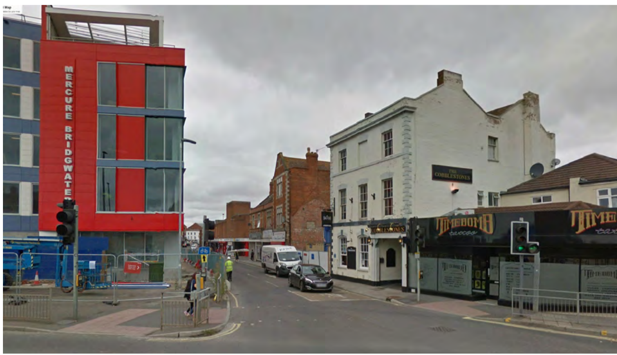
VIEW 01: EAST GATE LOOKING DOWN EASTOVER - EXISTING CONDITION
