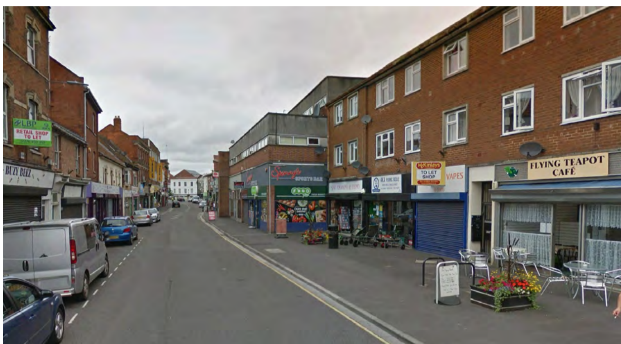
VIEW 02: CENTRAL EASTOVER LOOKING TOWARDS THE BRIDGE - EXISTING CONDITION
